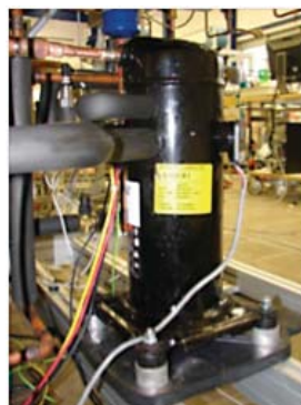
ZHW Scroll-kompressor for inverterdrift
